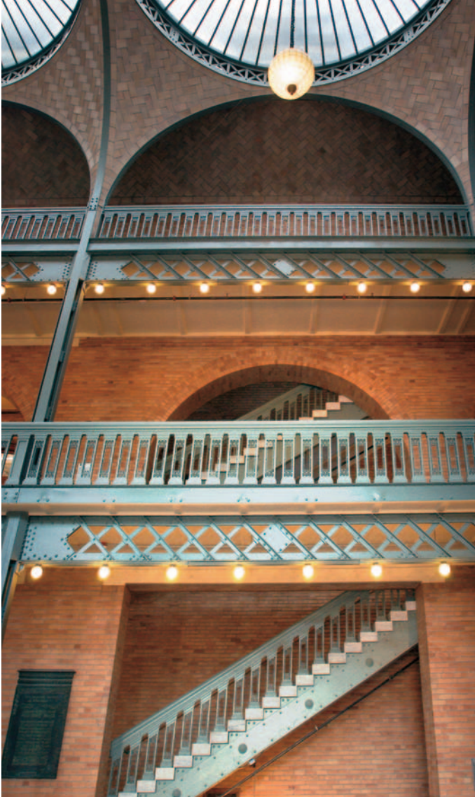
Hearst Memorial Mining Building's Memorial Gallery features skylights and arches decorated with Guastavino tiles, an early method of fireproofing.
