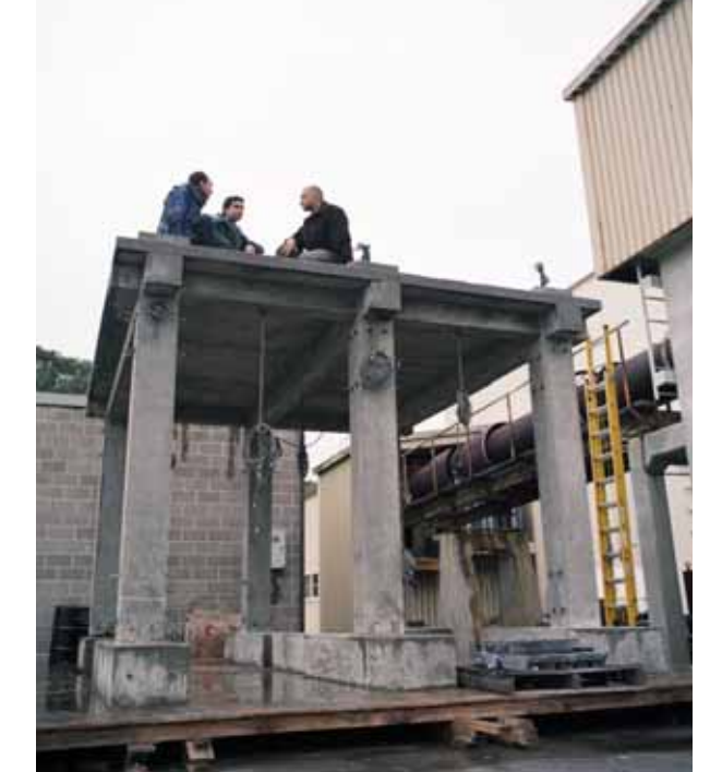
Packing some 95,000 pounds, this specimen is one of the largest and bulkiest ever tested on a shake table. Once hoisted onto the table, the team added a full-scale interior masonry wall, 80 sensors, and 150 strain gauges to measure the stresses and forces endured during months of testing.
