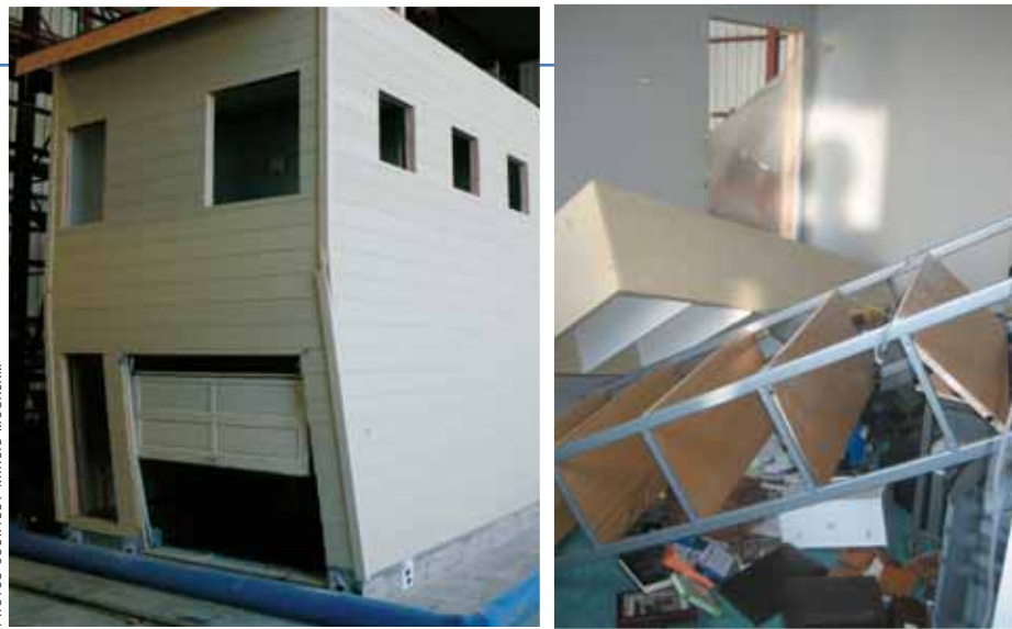
An 8.0 earthquake simulated on the shake table at Berkeley's Earthquake Simulator Lab was featured on NBC-TV's "Dateline" in May. Following the tests, the replica of a pre-code "soft-story" San Francisco home sustained structural damage, and unsecured furnishings on the second story came crashing to the floor.
