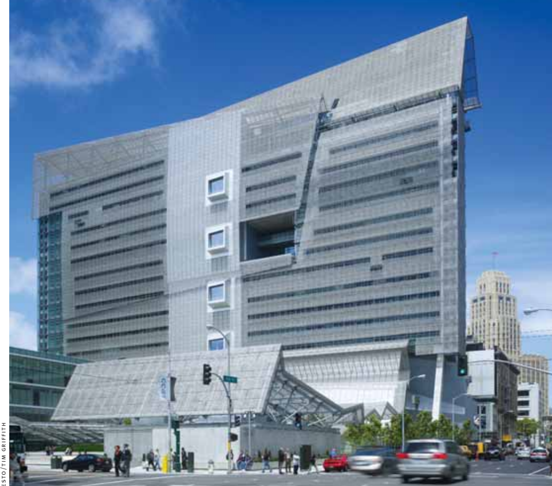
The San Francisco Federal Building features both manual windows at desk level and motorized windows at a greater height. From the building's southeast side, window panels flip up to a 90-degree angle to provide occupants a vista of San Francisco's SOMA district.
