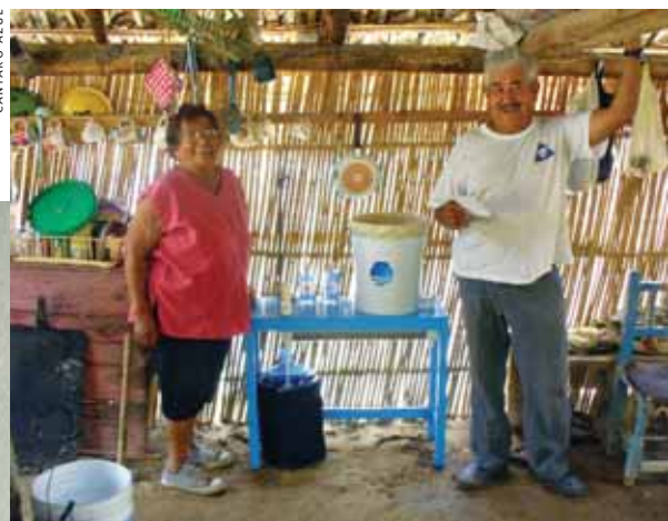
ABOVE: This Los Dolores family purifies a full day of drinking water in five minutes with their user-friendly water disinfection system, known as la mesita azul for the blue table it is mounted on.
