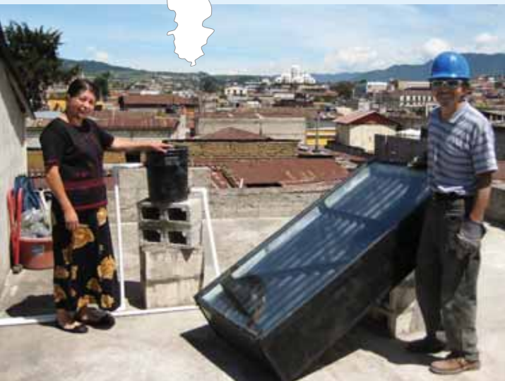
Mama Coney (left) and husband Papa Carlos demonstrate the water heater on the roof of their home in Xela, one of the households testing the CalSolAgua prototype. The unit uses a black sheet-metal absorber covered with glass to heat water supplied by a city pipeline.
